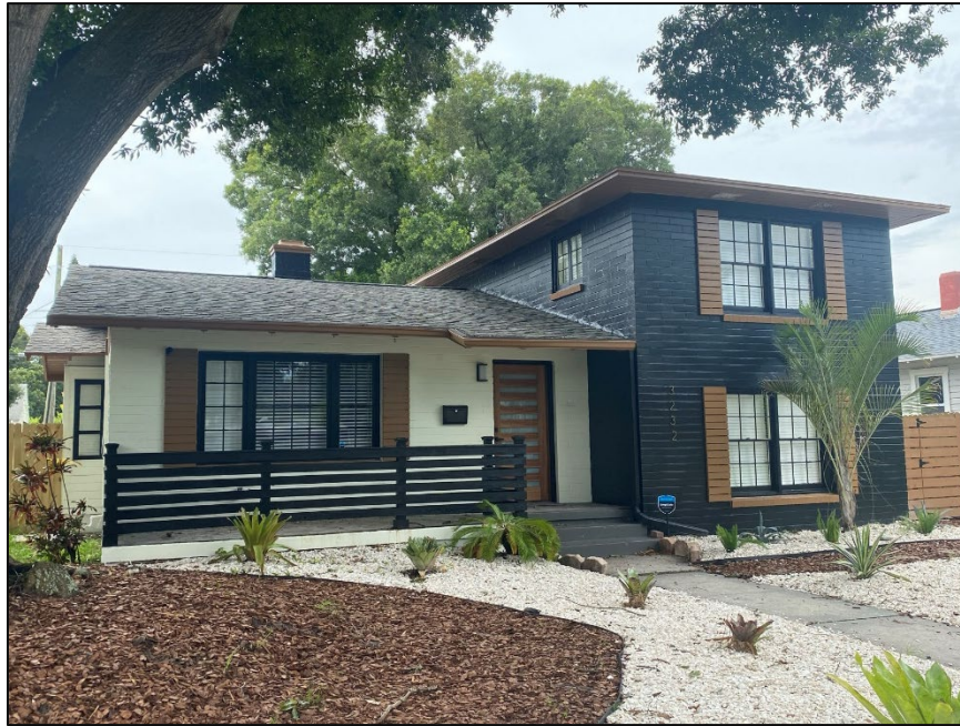
Figure 4: Staff photograph of subject property, August 16, 2021
