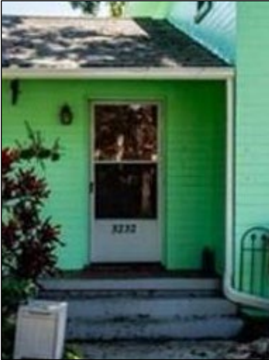
Figure 8: Previously-existing door and storm door (image from 2020 Coldwell Banker listing)
