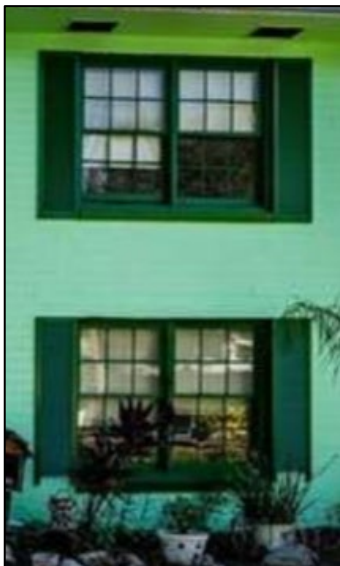
Figure 5: Louvered shutters at subject property prior to 2020 (not original; application photo)
