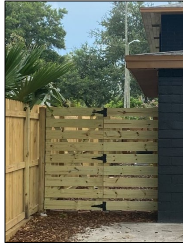
Figure 13: Rear side fence and gate
