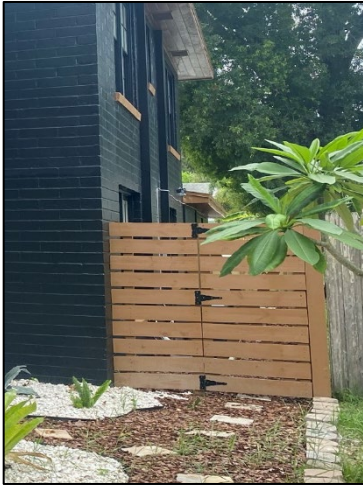
Figure 12: Front right side fence and gate
