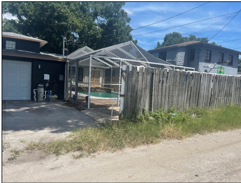
Figure 14: Existing rear fence at subject property
